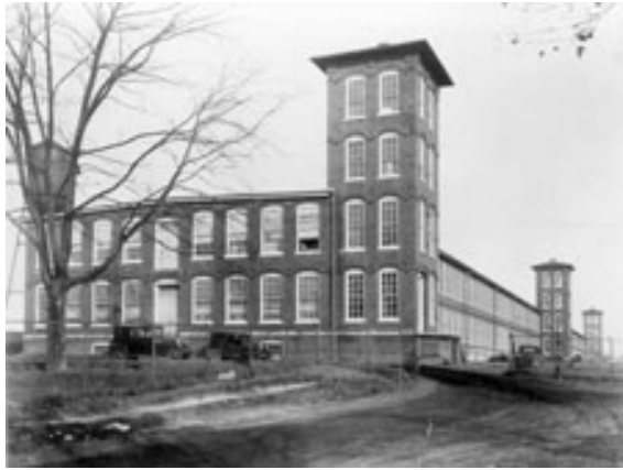
Erwin Mills, from Main St. c. 1920.
